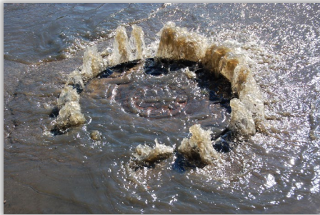
Sanitary Sewer Overflow
